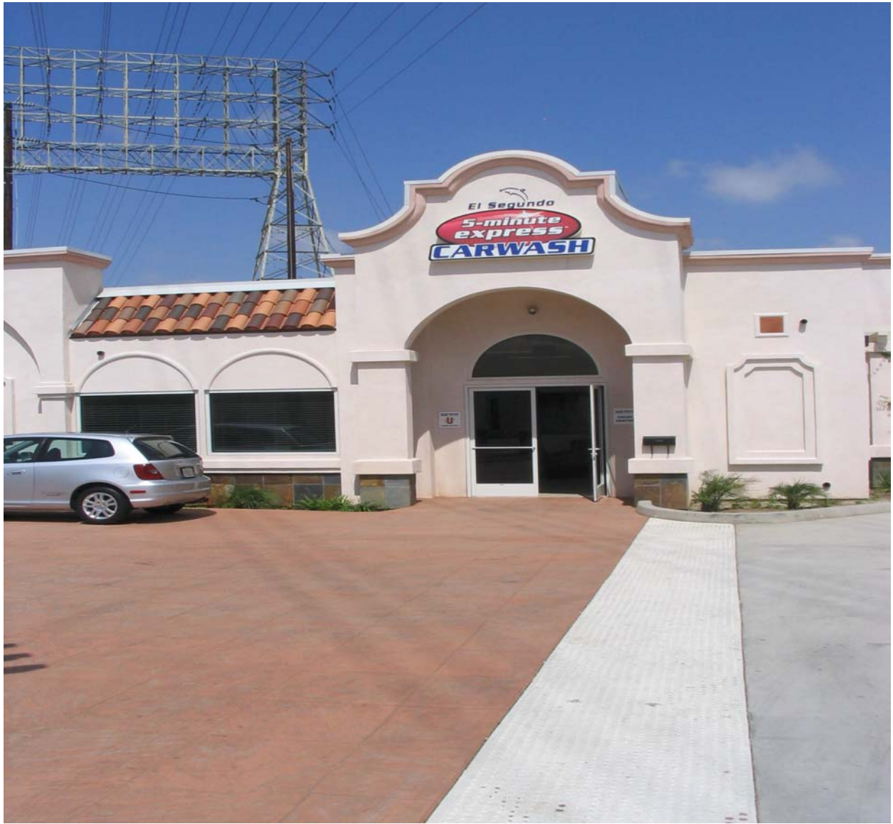
Entrance to Offices Inside Tunnel Building
